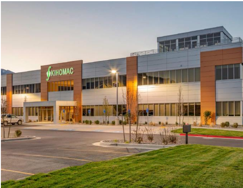
KIHOMAC at East Gate Business Center
