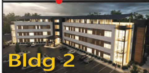
Bldg 2 UNDER CONSTRUCTION
